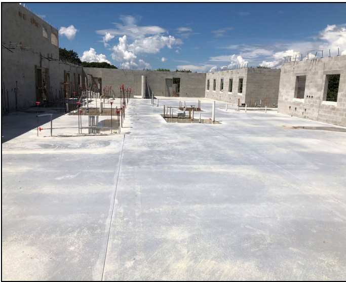
Apollo Beach Fire Station #29 Under Construction
