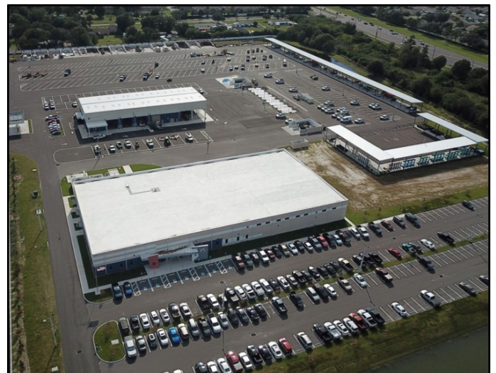
Consolidated and Hardened Maintenance Facility – South Service Unit
